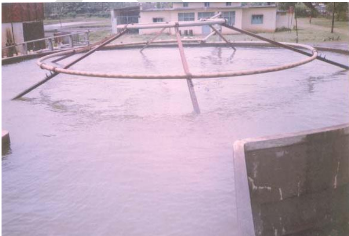
Figure : . Top view of a Chinese type of circular breeding tank, with an overhead shower(above & below).
